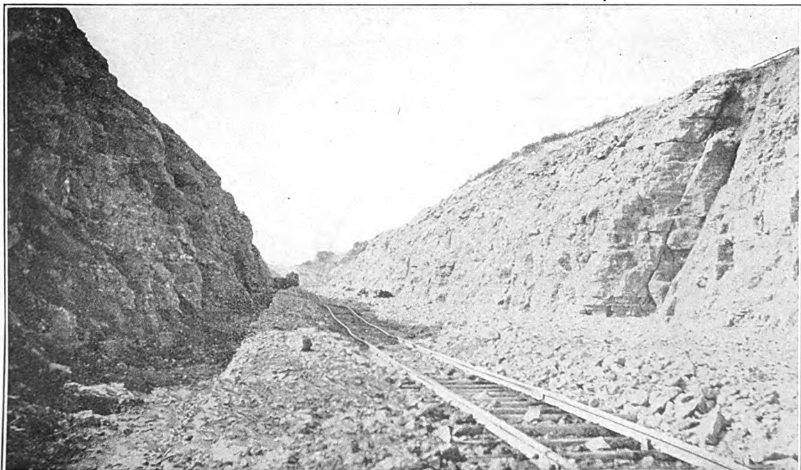
Fig. 4—Rock Cut Near Browns, Ia., Maximum Depth 55 ft.
