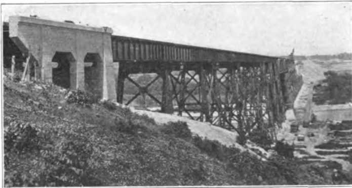
General View of the Des Moines River Viaduct
