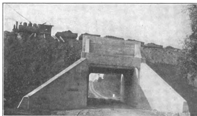
A Special Type of Highway Under Crossing, Securing a Short Barrel by Use of High Parapet Wall
